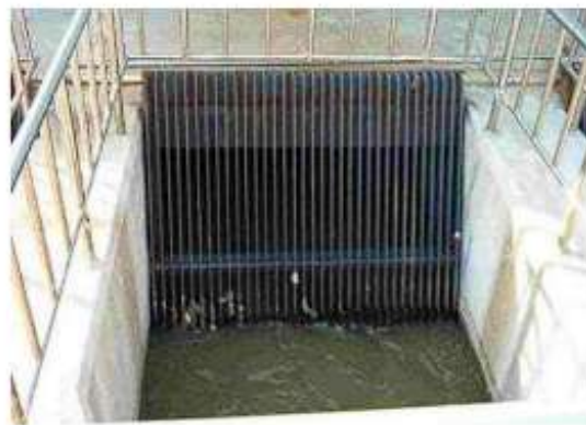
Gambar 2.7 Coarse Screen
