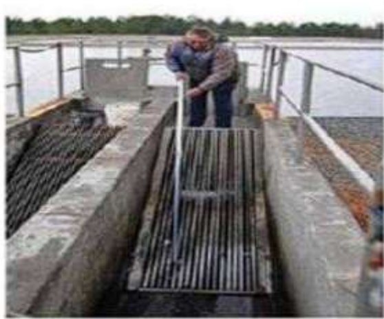
Gambar 2.8 Manual Bar Screen
