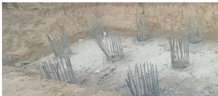
Gambar 2. 3 Bored Pile
