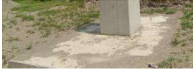
Gambar 2. 4 Pile Cap
