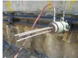
Gambar 8. 12 Stressing ground anchor
