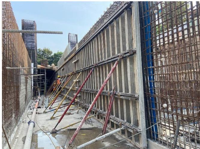
Gambar 7. 22 Pemasangan Bekisting Dinding
