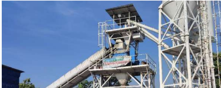
Gambar 10.14. Persiapan Batcing Plant
