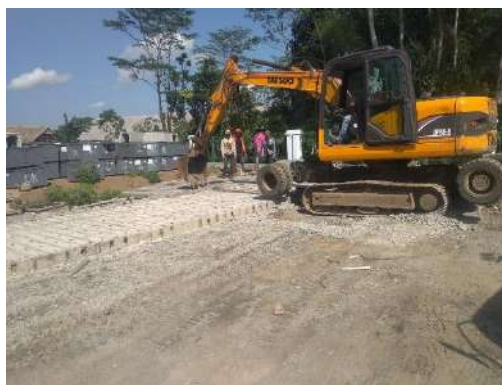
Gambar 4.7. Excavator on The Wheel
