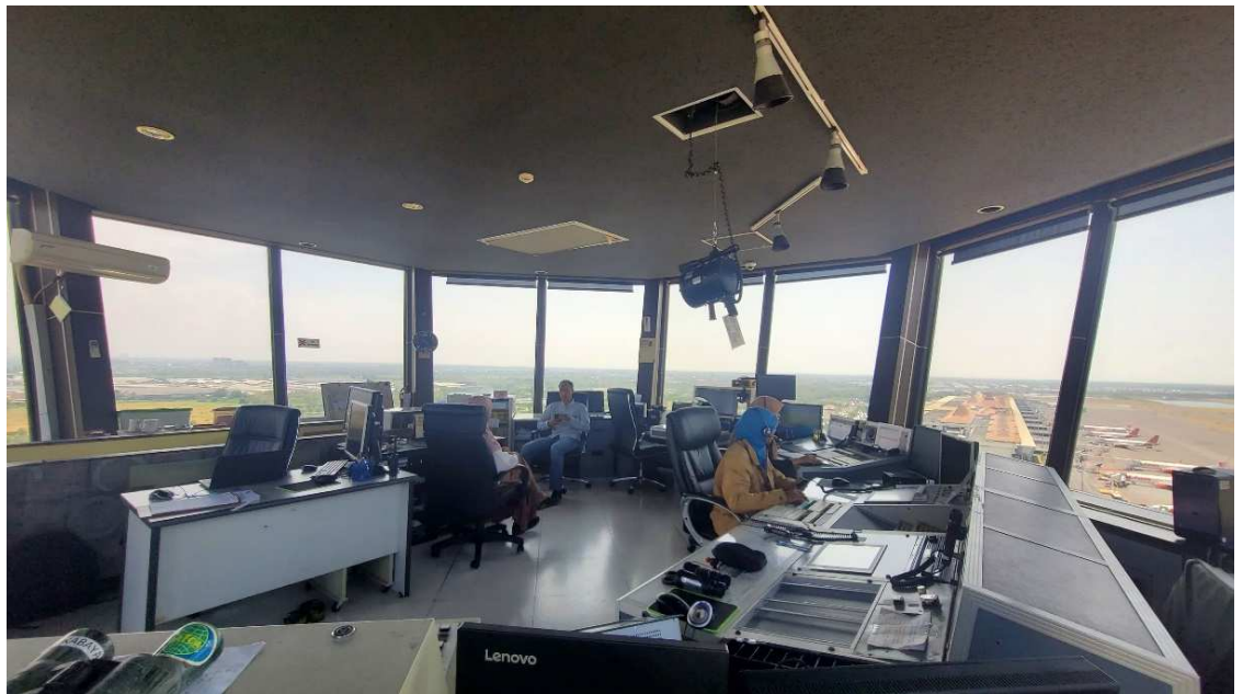
Ruang Tower ATC AirNav Surabaya
