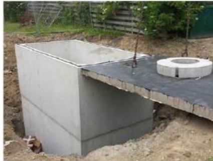
Gambar 2.26 Reservoir Beton Cor
