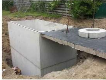
Gambar 2. 15 Reservoir Beton Cor
