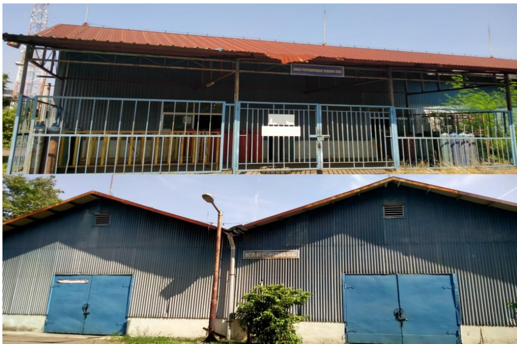
Gambar 1.3 Warehouse PT Boma Bisma Indra Pasuruan
