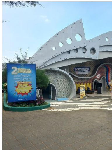
Gambar 2.44 Gedung Hanoman Bioskop Dome 3D
