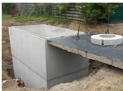
Gambar 2. 11 Reservoir beton cor
