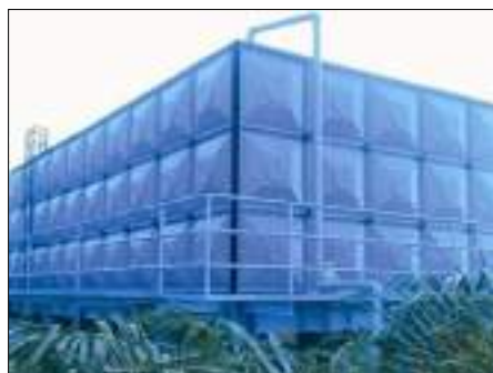
Gambar 2. 26 Reservoir Fiberglass
