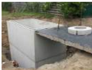
Gambar 2. 25 Reservoir Beton Cor
