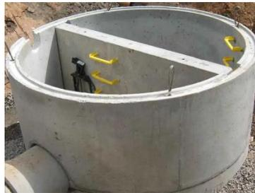
**Gambar 2.17** Reservoir Beton Cor
