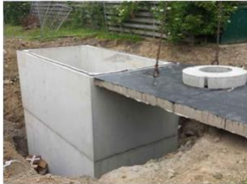
Gambar 2.20 Reservoir Beton Cor
