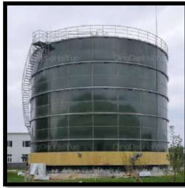
Gambar 2. 29 Reservoir Tanki Baja
