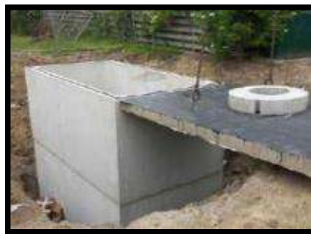
Gambar 2. 30 Reservoir Beton Cor
