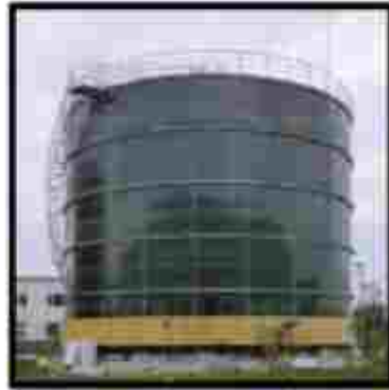
Gambar 2. 20 Reservoir Tangki Baja
