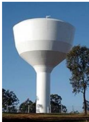
Gambar 2. 22 Elevated Reservoir (Menara Reservoir)
