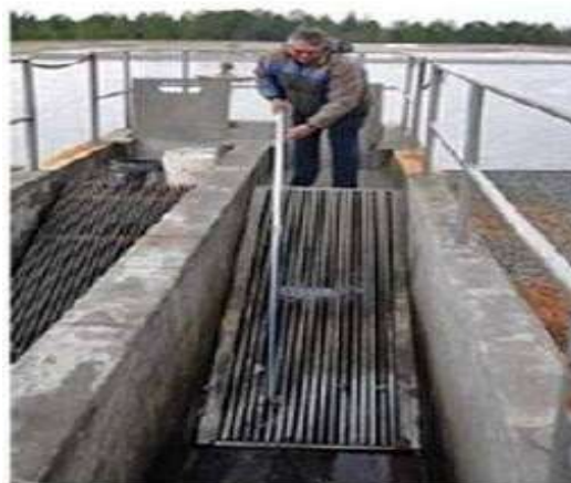
Gambar 2.2 Manual Bar Screen
