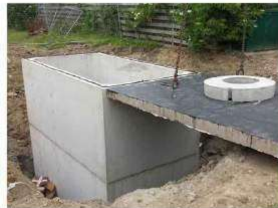
Gambar 2. 21 Reservoir Beton Cor
