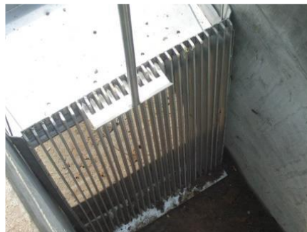
Gambar 2. 1 Manual Bar Screen
