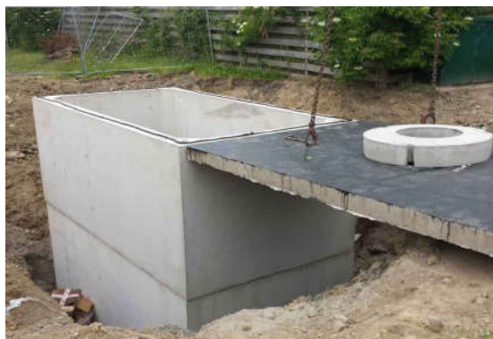
Gambar 2. 18 Reservoir Beton Cor
