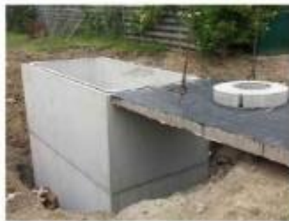
Gambar 2.11 Reservoir Beton Cor
