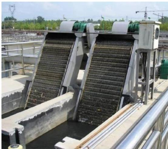
**Gambar 2.3** *Mechanical Bar Screen*
