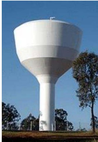
Gambar 2.25 Elevated Reservoir (Menara Reservoir)
