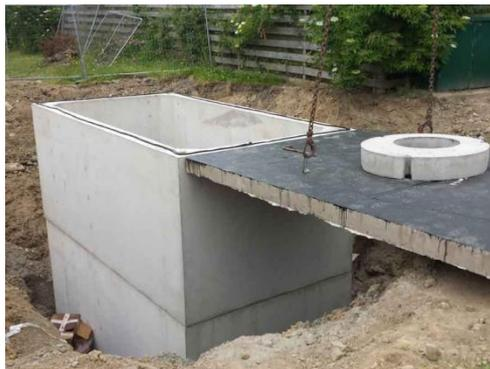
**Gambar 2. 22 Reservoir Beton Cor**
