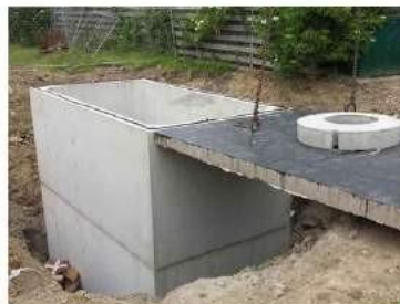
Gambar 2. 4 Reservoir Beton Cor
