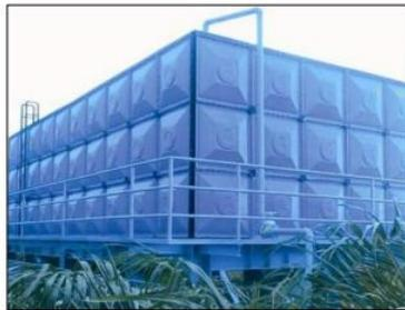
**Gambar 2. 24** Reservoir Fiberglass
