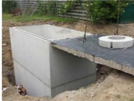
**Gambar 2. 23** Reservoir Beton Cor
