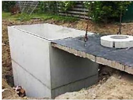
**Gambar 2.9** Reservoir Beton Cor
