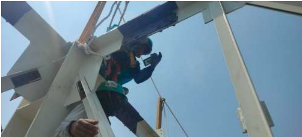
Gambar 6. 14 Pekerjaan Second Touch Up Material
