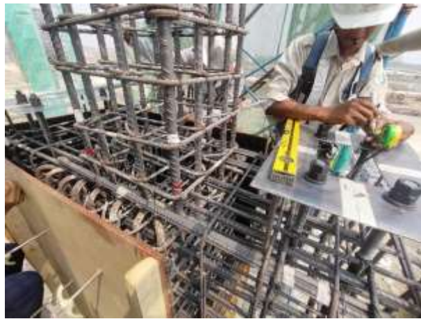
Gambar 6. 3 Pekerjaan Formwork Angkur
