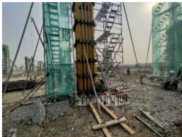
Gambar 4. 3 Formwork Kolom
