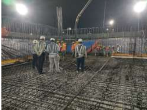
Gambar 4. 12 Proses Pengecoran Beton Integral
