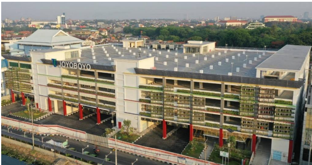
Gambar 1.4 Gedung Park and Ride Terminal Intermoda Joyoboyo Sumber : dishub.surabaya.go.id, 2023
