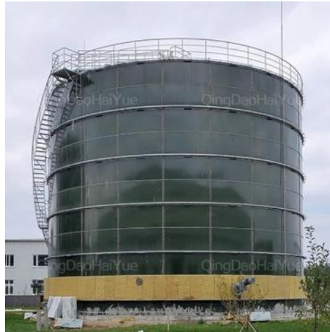
Gambar 2. 16 Reservoir Tanki Baja
