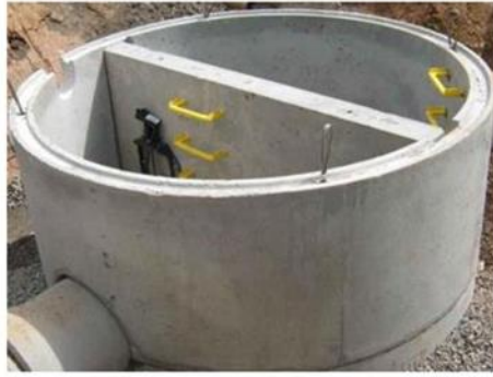
Gambar 2. 17 Reservoir Beton Cor
