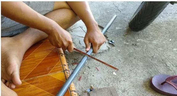
**Gambar 9.** Memotong Pipa Paralon
