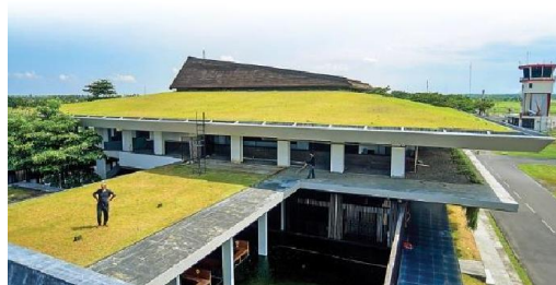
Gambar 2.15 Roof Garden Bandara Banyuwangi Sumber: Google Images , 2020.
