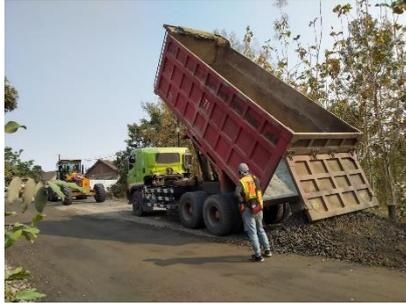
Gambar 8.8 Dropping Agregat Kelas A
