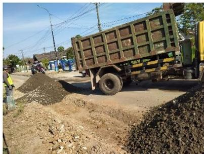
Gambar 8.3 Dropping Agregat Kelas A
