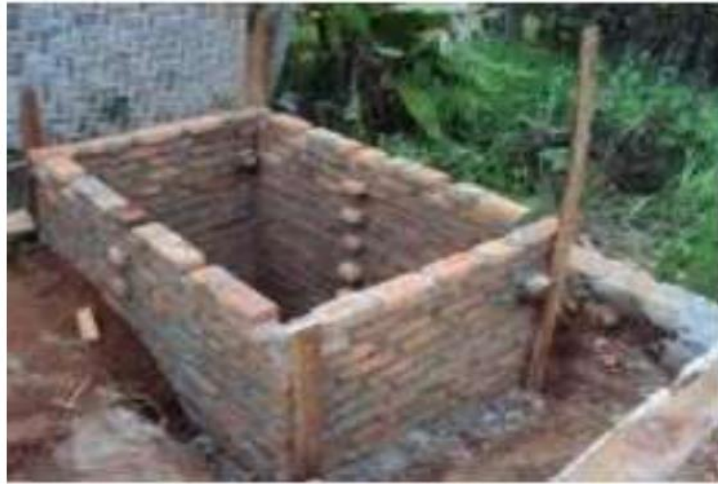
Gambar 2. 38 Reservoir Pasangan Bata
