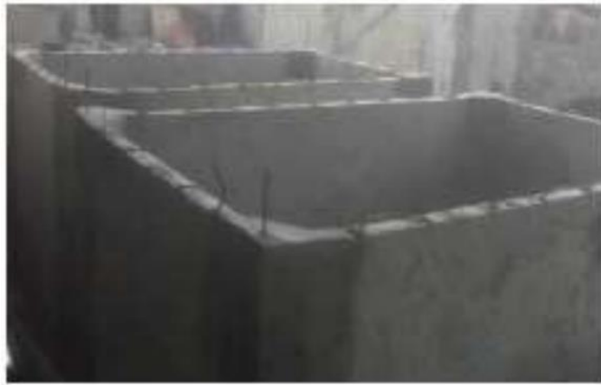
Gambar 2. 37 Reservoir Beton Cor
