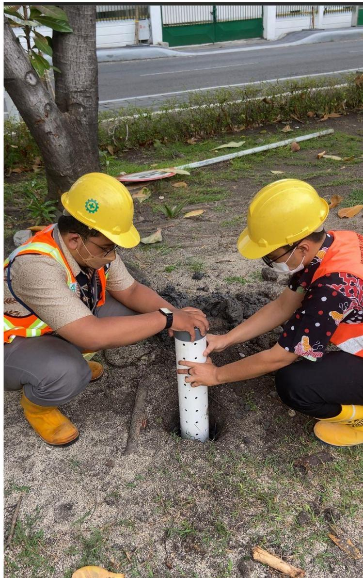
**Gambar 2.3.** Pemasangan proyek Lubang Reseapan Biopori
