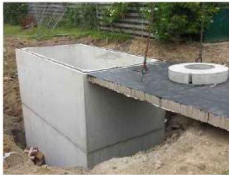
Gambar 2. 24 Reservoir Beton Cor
