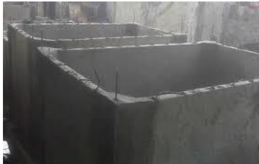
Gambar 2. 20 Reservoir Beton Cor
