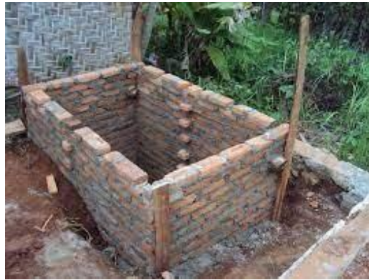
Gambar 2. 22 Reservoir Pasangan Bata
