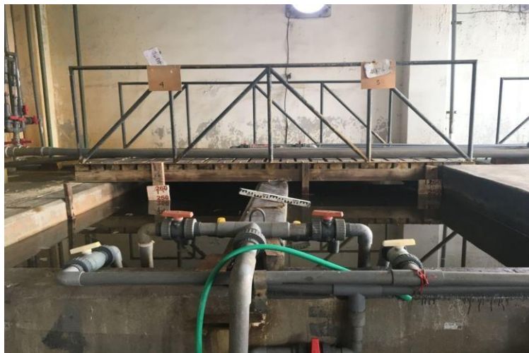
Gambar 2. 15 Bak Larutan Tawas
