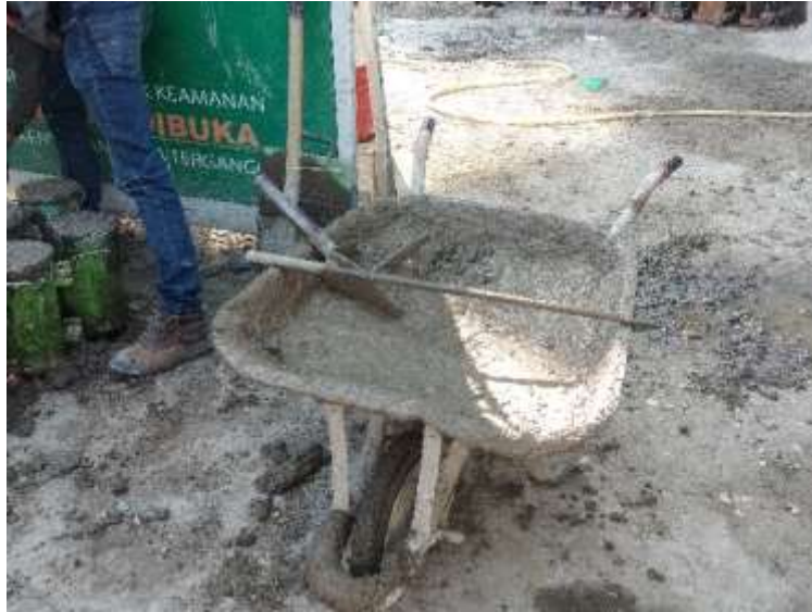
Gambar 2.1 Beton Ready Mix
