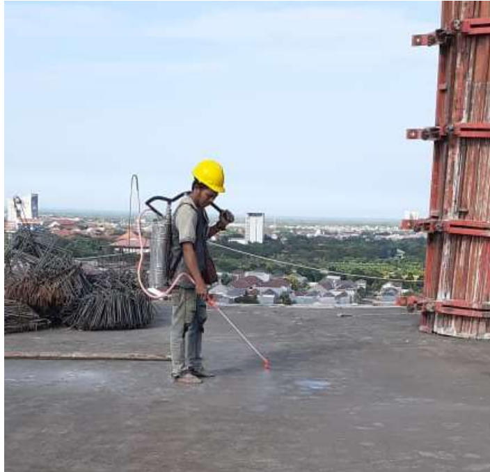
Gambar 2.6 Curing Beton
