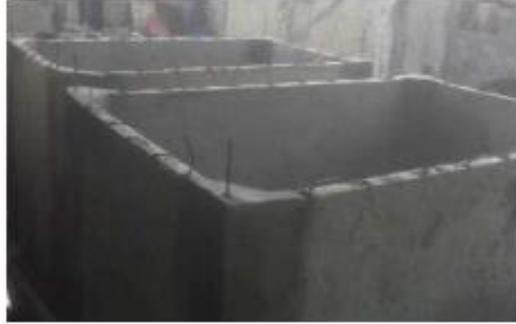
*Gambar 2.30 Reservoir Beton Cor*
