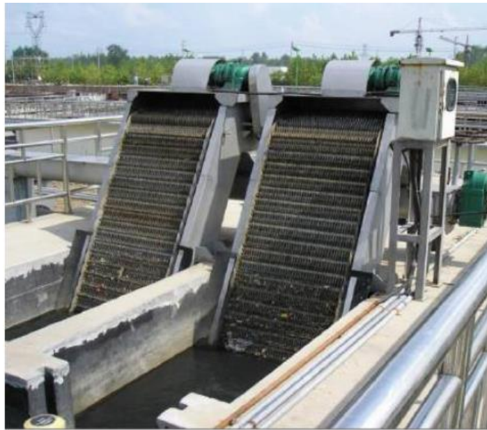
Gambar 2. 3 Mechanical Bar Screen
