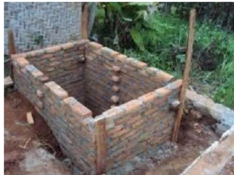
Gambar 2. 23 Reservoir Pasangan Bata
