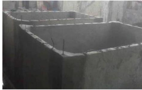
Gambar 2. 22 Reservoir Beton Cor
