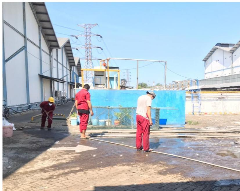
Gambar 5. 11 Pembersihan Perforated Tubing
