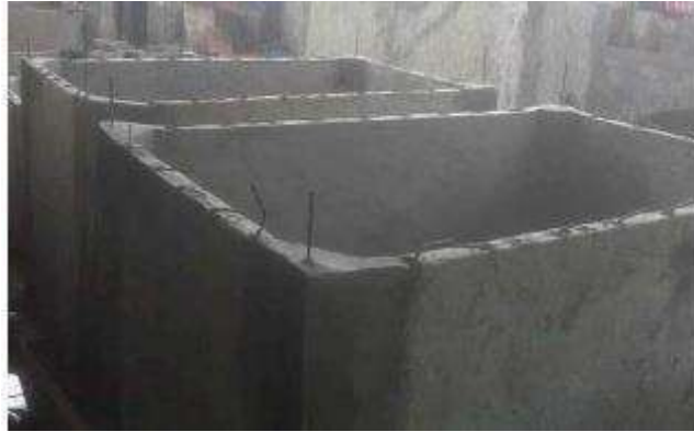
Gambar 2. 30 Reservoir Beton Cor
