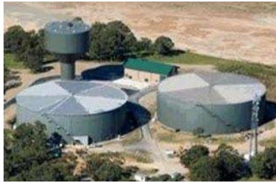
Gambar 2. 29 Reservoir Tangki Baja
