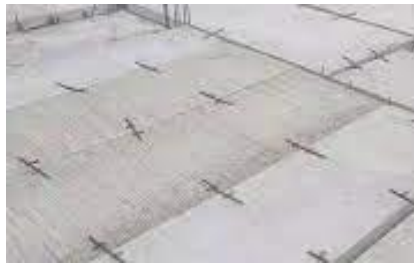
Gambar 2.6 Atap Dak Beton
