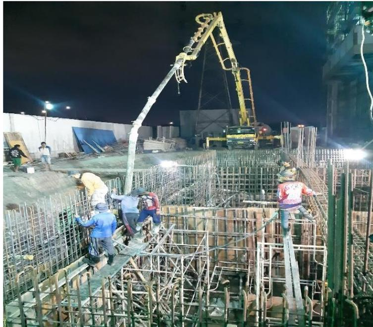
Gambar 2. 7 Truck Concrete Pump
