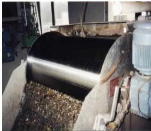
Gambar 2. 3 Rotary Drum Fine Screens
