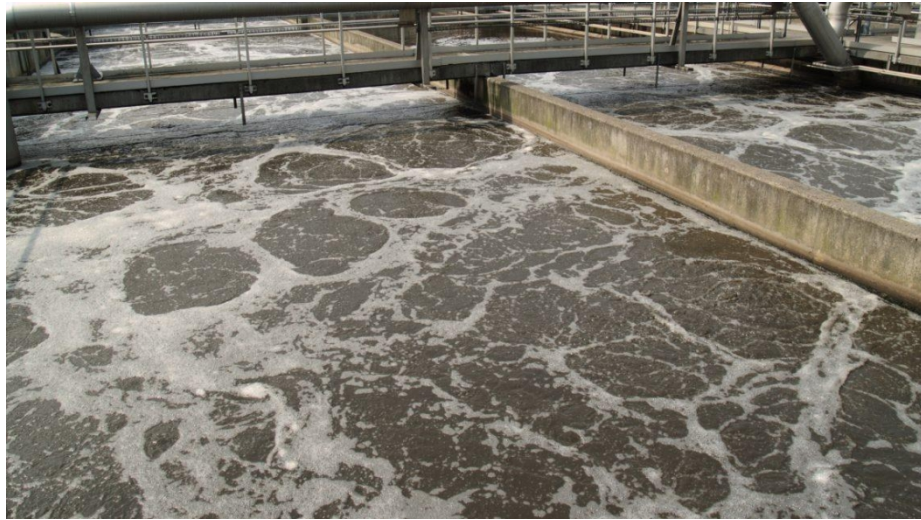
Gambar 2.12 Aerated Activated sludge
